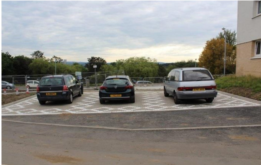
Image 2: Permeable paving serving car parking areas
