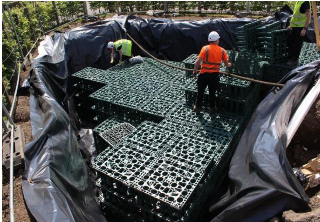
Image 1: Geocellular structure under construction
