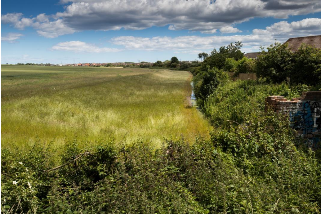
Figure 4: Upstream attenuation along the Forest Hall Letch in a two stage channel, which reduces downstream flooding and provides new habitat and enhances biodiversity in this area
