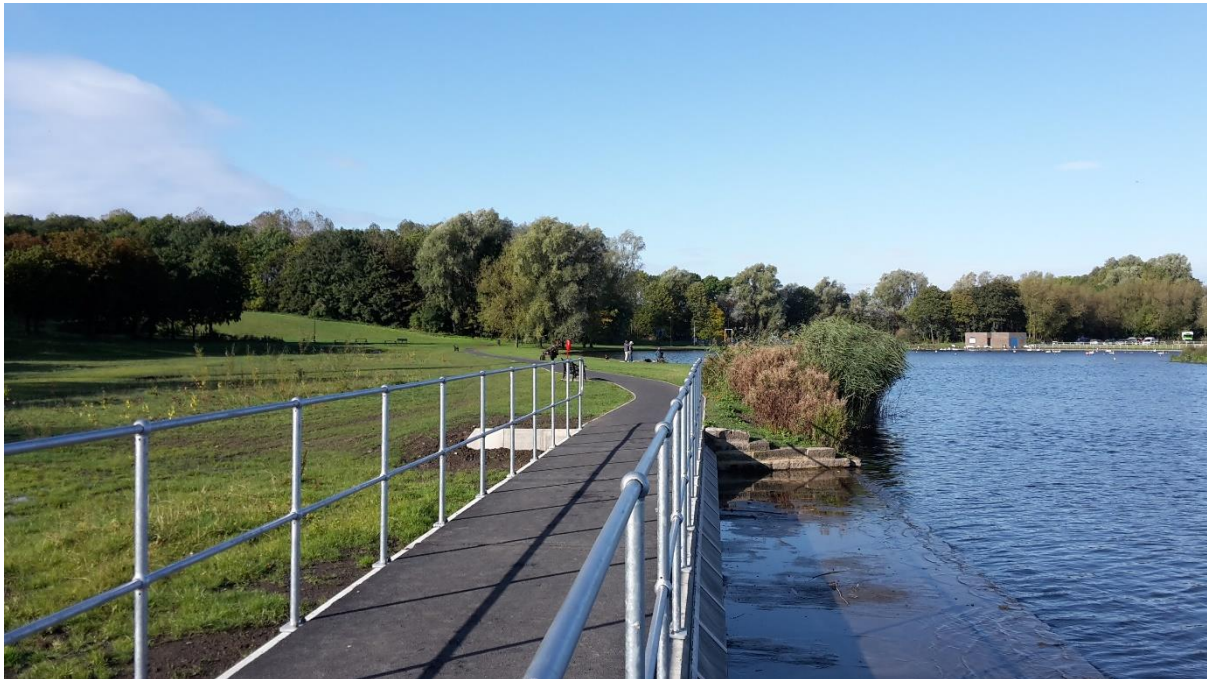
Figure 8: New pathways and a bridge over the weir are located adjacent to the attenuation area. These are part of an improved pedestrian route, which enhances the recreational opportunities within the Killingworth Lakeside Park.
