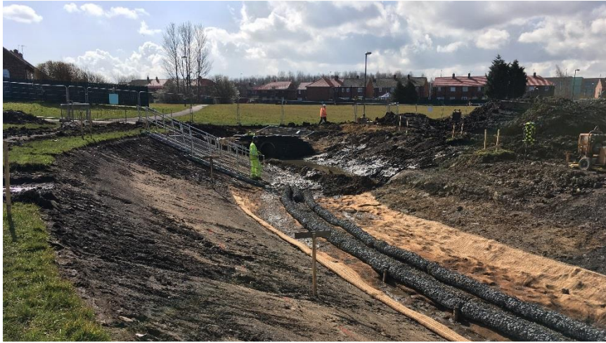
Image Description – Attenuation Basin (daylighting) under construction at Toner Avenue School
