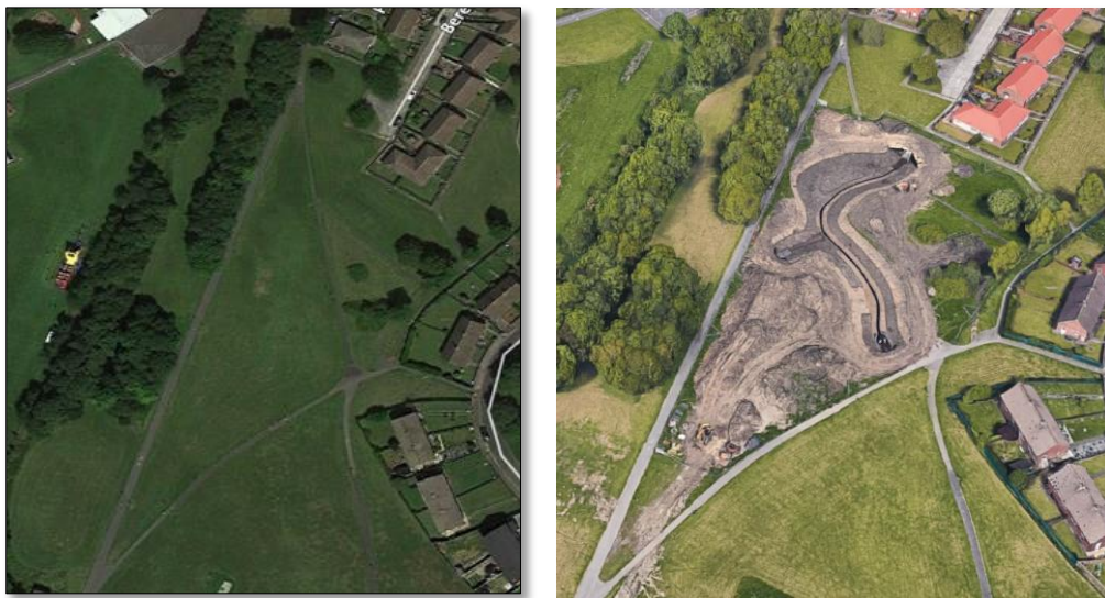
Aerial Images showing Bede Burn daylighting section pre construction (left) and during construction (right)
