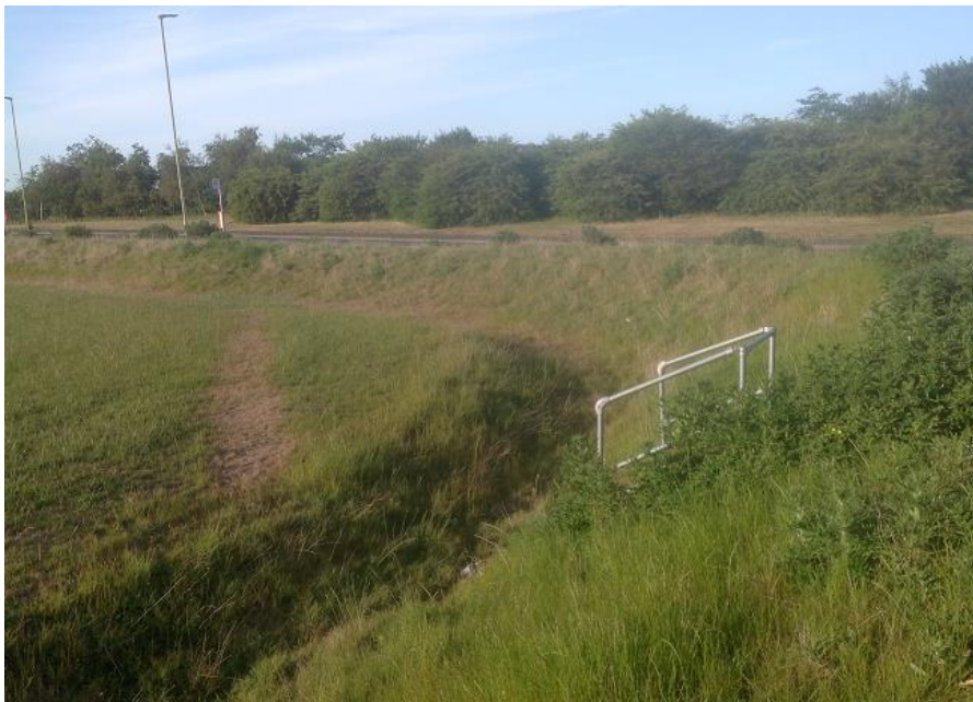
Image Description- Completed Bund/Swale at Lukes Lane
