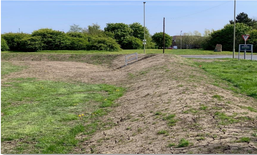
Image Description – Bund/Swale under construction at Lukes Lane
