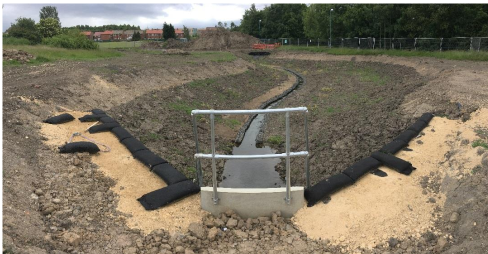
Image Description – Attenuation Basin (daylighting) under construction at Toner School
