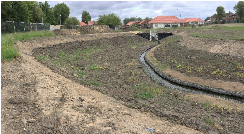
Image Description – Attenuation Basin (daylighting) under construction at Toner Avenue School
