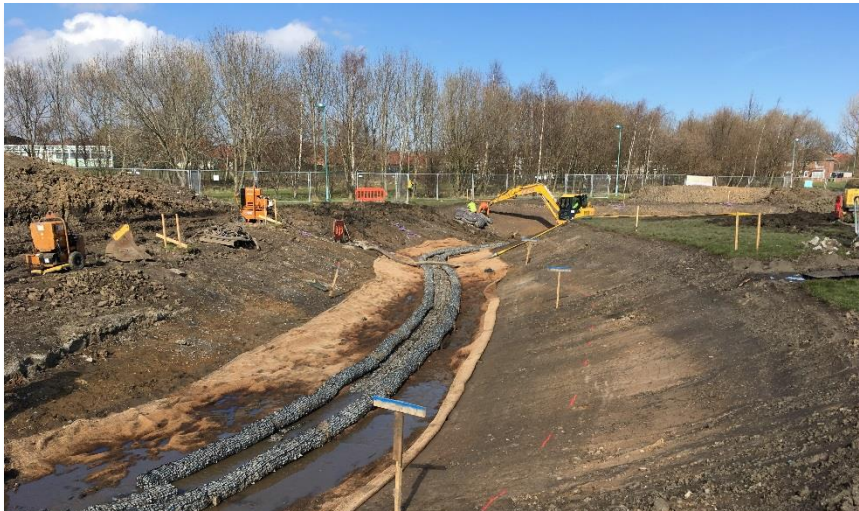
Image Description – Attenuation Basin (daylighting) under construction at Toner Avenue School
