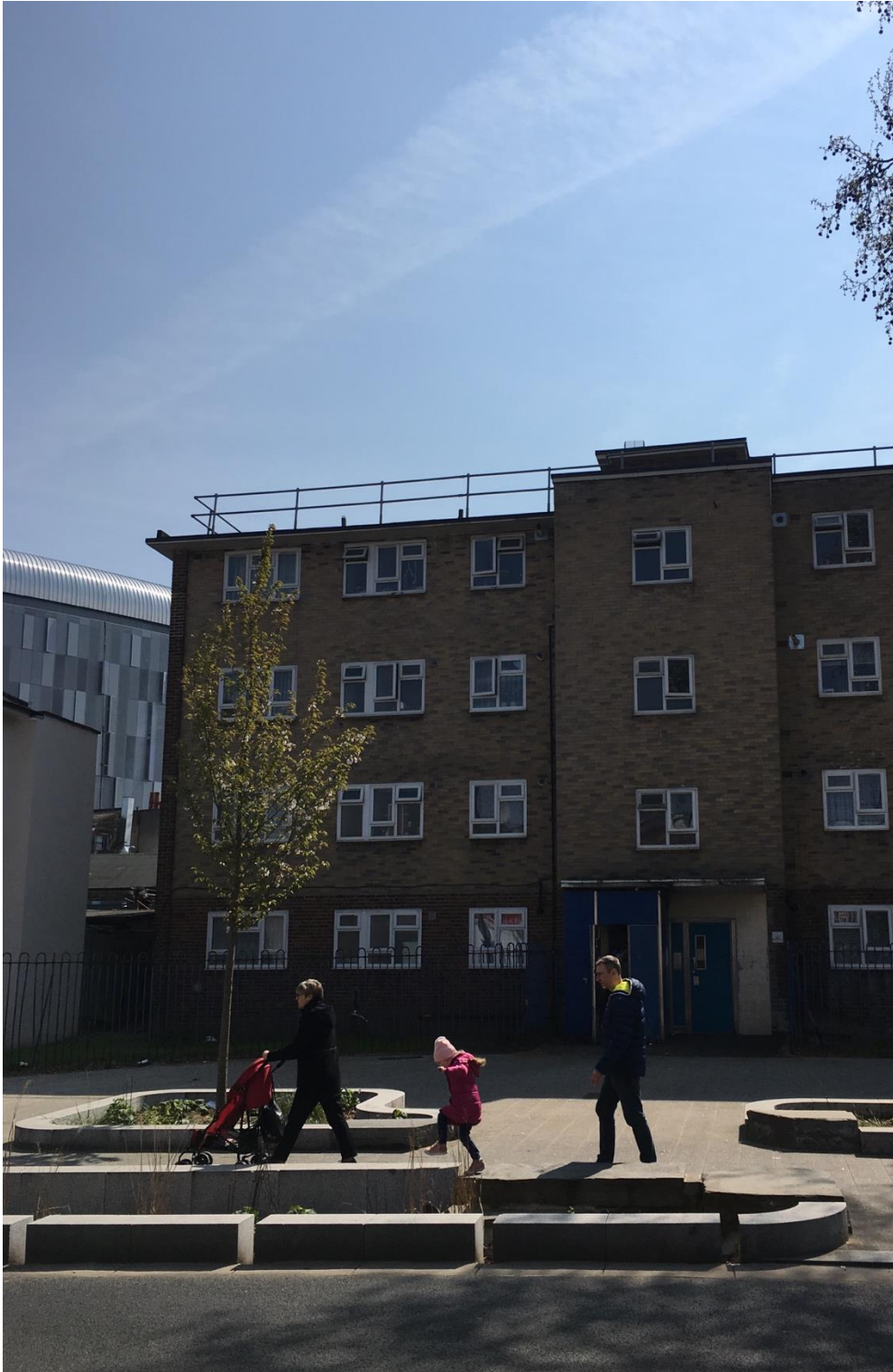
Playable SuDs with Raingarden stepping stones (before planting established)
