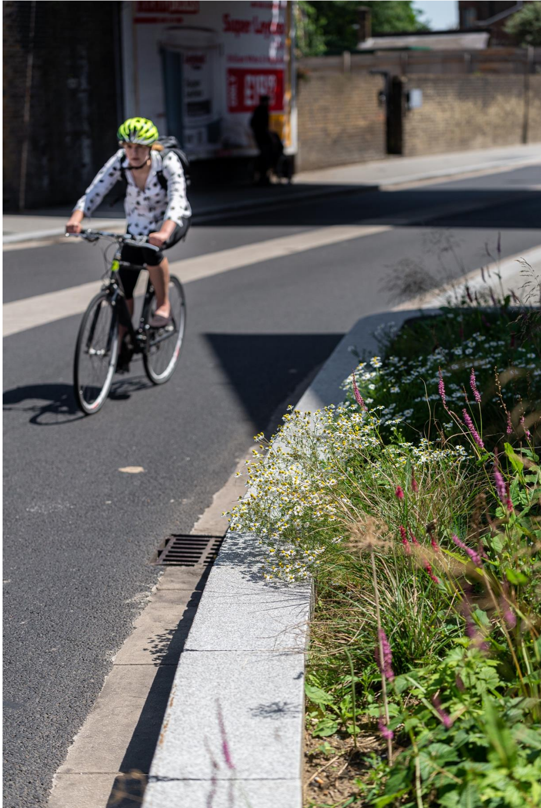
Modal change through narrowing the road and adding roadside raingardens and planting
