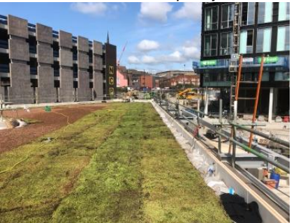
Green roof installation on 'The Kiosk' building
