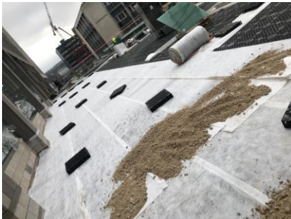
Installing water flow reducing layer to Level 50
