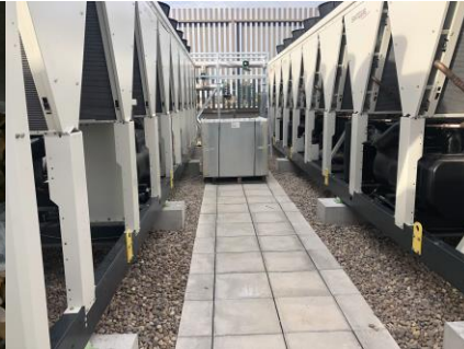
Paving slab maintenance walkway on Level 60
