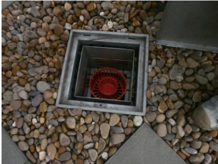
Restrictor Chamber & RWO Level 60
