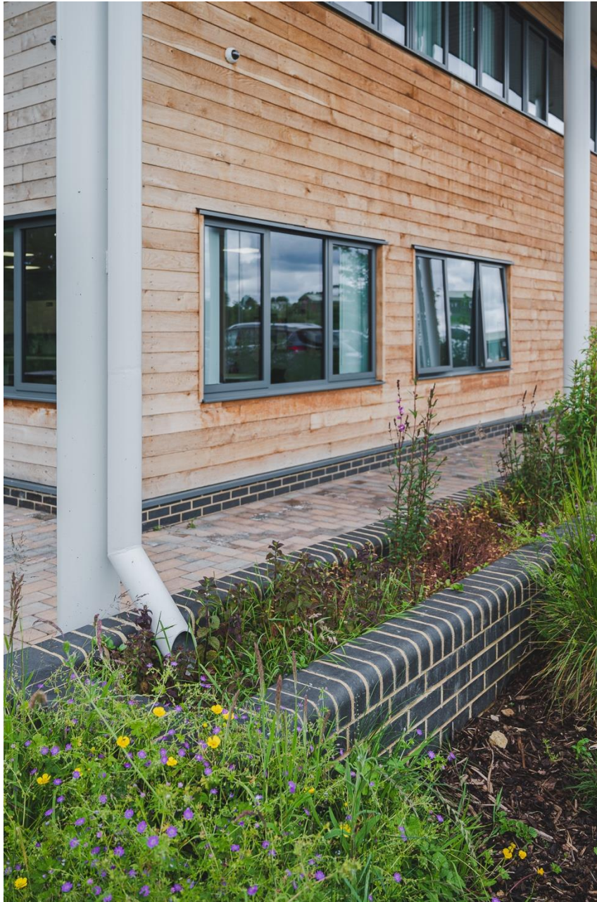
Raised wetland feature and one of a number of rainwater pipe inlets.
