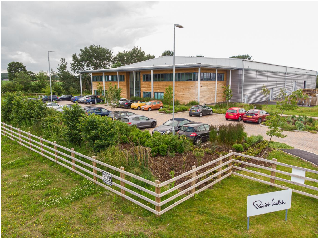
View of the car park and front of building
