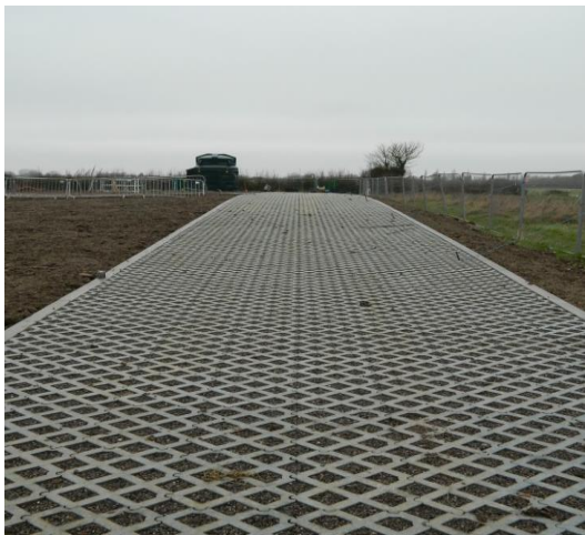
Completed section of permeable paving access road
