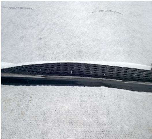
Geocomposite drainage install (example)
