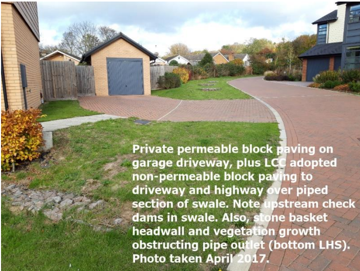
Highway adopted non-permeable block paving, abutting permeable block paving serving private driveway (householder responsibility). Note grass filter strips, flow conveyance swales and check dams, plus different patterns in block paving with slender concrete edging indicating change in responsibility. Photo taken April 2017.
