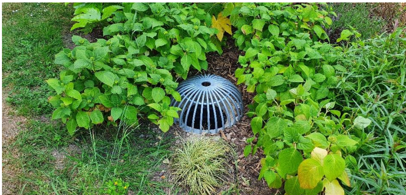
Fig 1: Custom made domed gully cover
