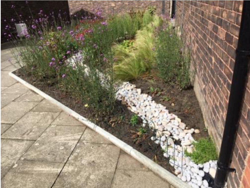
Rain garden – during construction
