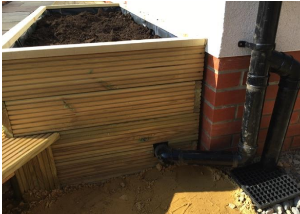
Downpipe connection to raised bed & overflow
