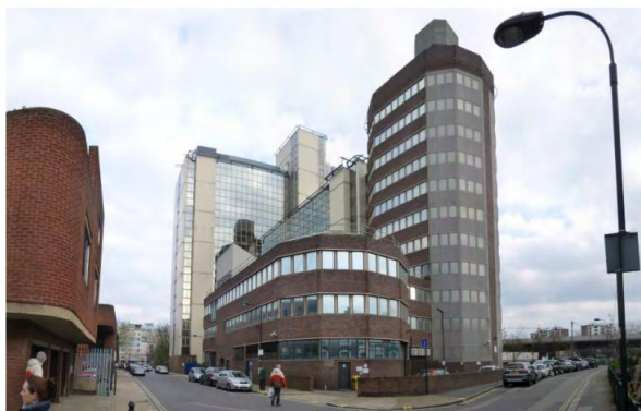
Thames Tower from intersection of Black's Road and Angel Walk
