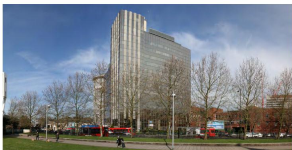
Landmark House from St. Paul's Green
