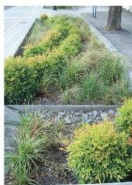
Figure 31.5 Bioretention planter in street
