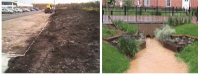
Figure 13.1 Mud being spread by vehicles or from soil surfaces onto permeable paving. Figure 13.2 Muddy runoff washing into SuDS.
