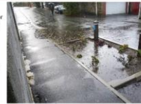
Incorrect soil mix, does not drain sufficiently
