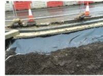
Bioretention system filled with specified engineered soil mix
