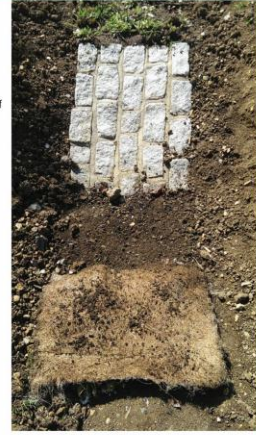
Figure 23.12 'Outlet' blocking flow along the SuDS management train
