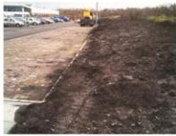
Figure 13.1 Must being spread by vehicles or from soft surfaces onto permeable paving
