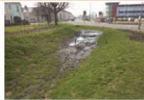
Erosion at base of bank falling due to lack of time to establish
