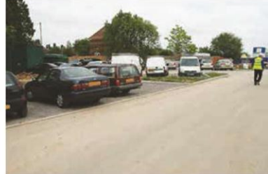
Figure 12.2 Sacrificial sub-base layer allows use of permeable sub-base for parking during construction
