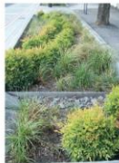
Figure 31.5 Bioretention planter in street
