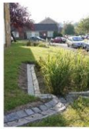
Figure 31.1 Small domestic rain garden
