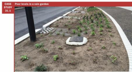
Figure 31.19 Level of soil above the level of inlets from road
