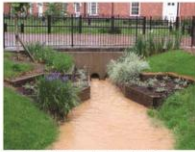
Figure 13.2 Muddy runoff washing into SuDS
