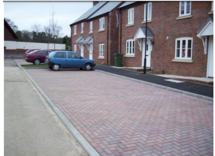
Permeable pavement with infiltration close to house foundations
