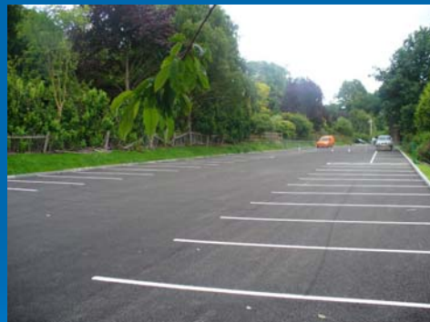
Porous asphalt to car park – Little Eaton Recreation Ground
