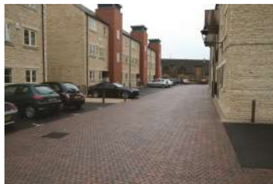
Figure 1 Use of SuDS in Stamford in a floodplain and area of contamination (EPG Ltd)
