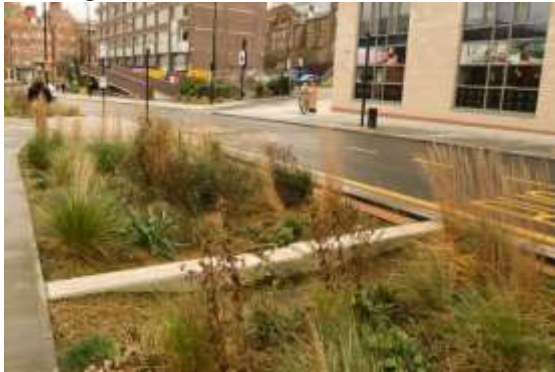
Figure 4 Use of check dams in a swale in the Grey to Green project in Sheffield
