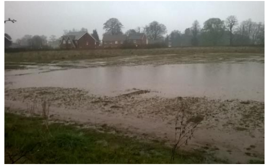
Half built swale but left as if complete (courtesy of Bob Haddon)
