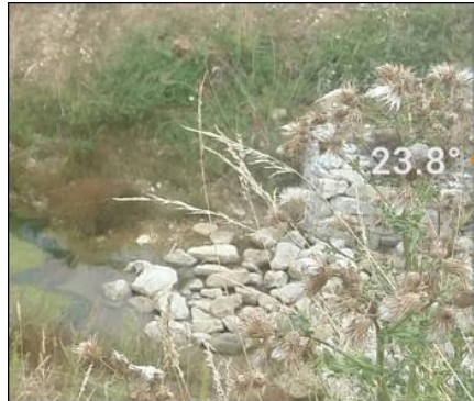
A collapsed structure creates a blockage that prevents water from leaving the feature
