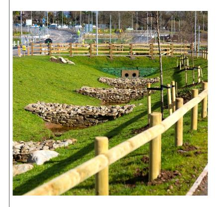
Swales were used to allow sheet flow of water from the highway and adjacent footway on the surface. The swales reduced the water pollution across the site.
