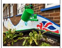
Watering can features were included on two of the planters to direct the roof runoff onto custom made miniature gabion baskets. This dissipates the water's energy and helps disperse the water evenly across the soils surface and avoids splashing. The gabions also ensure a safe solution for including cobbles, thus reducing the health and safety/vandalism risk within a school setting.
