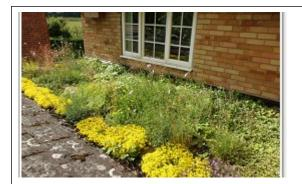
The house green roof: the flat garage roof was replaced with a green roof in 2010 (8.5m²), and provided a much improved view out of the window of the old office space in the house, until we were able to construct the garden office building. It also helps to regulate the temperature in the garage below.
