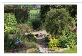
When the shallow basin in the rear lawn overtops, it flows through a dry stream bed feature to the rear of the garden, where there is a ditch forming part of the local surface water drainage system.
