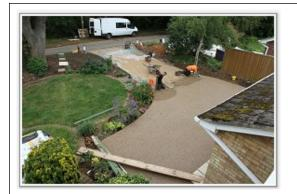
The permeable driveway under construction, with rain garden/hydration channel seen in the curved bed in the centre of the photograph.
