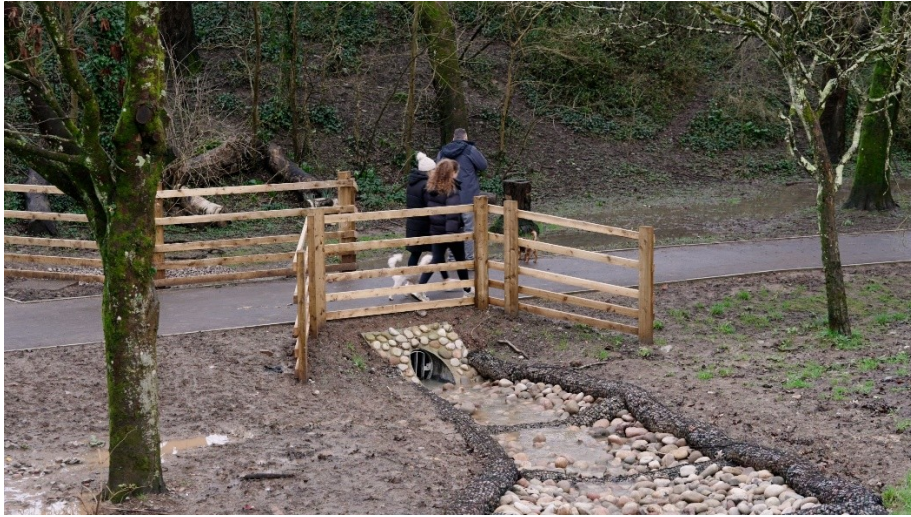
Cascade feature with erosion proofing
