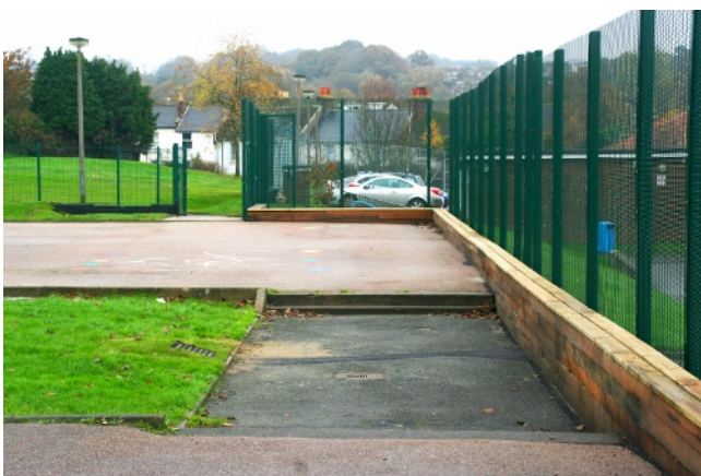
Figure 3: Timber seating wall converts an existing hard play area into a water large storage facility whilst providing added amenity for children.
