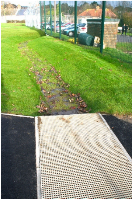
Figure 1: Bridge construction (before swale planting) allows shallow swale depth and grating surface intercepts path runoff.
