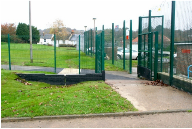
Figure 4: The recycled plastic slot weir is located adjacent to a gate, modified to retain stored water, and beyond the fence, the start of the timber sleeper storage wall (prior to planting).
